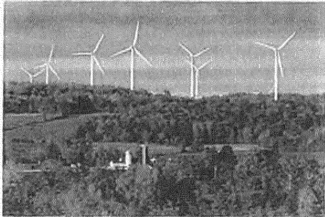
Photo courtesy of National Renewable Energy Laboratory (NREL), PIX 15249.
