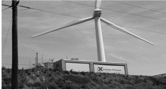
Xtreme Power KWP 1
