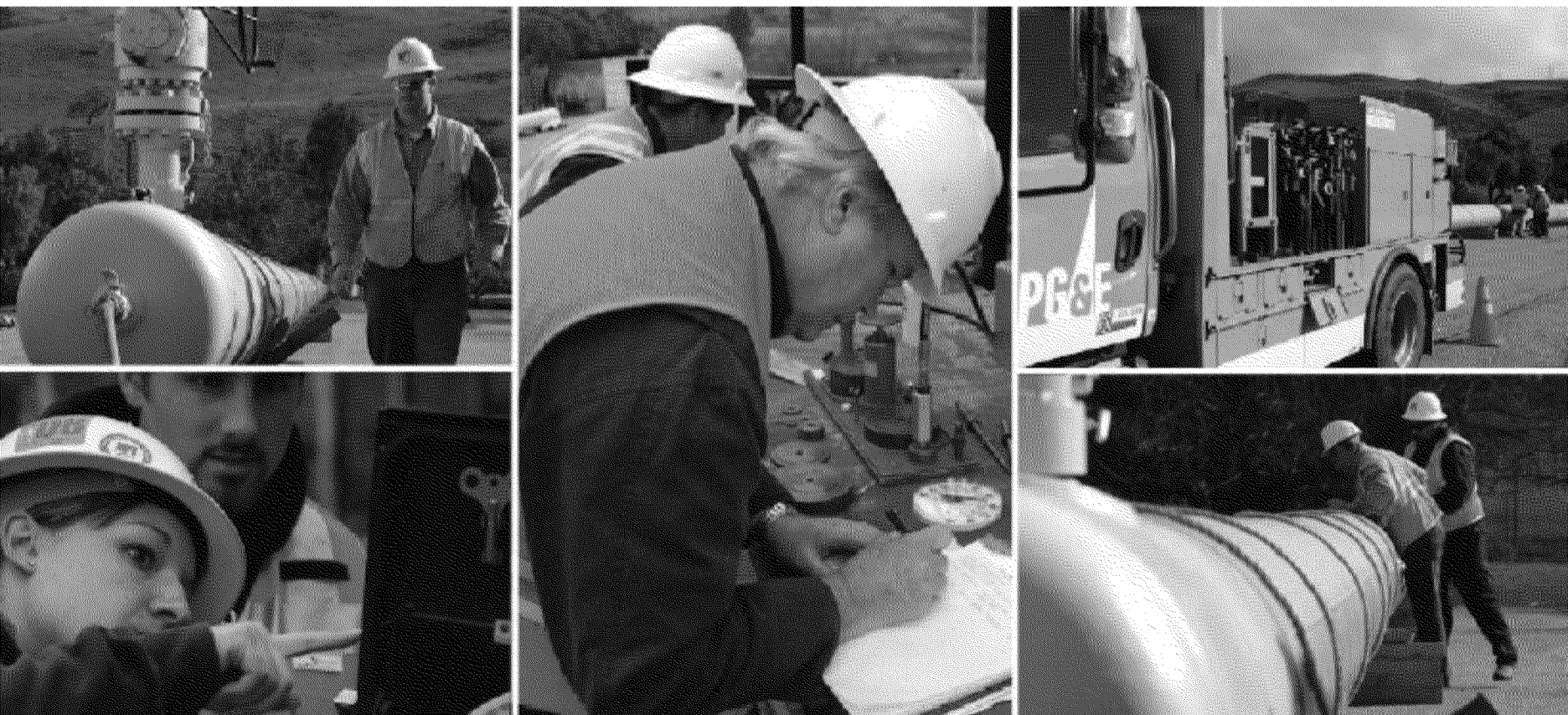
Pressure testing for the safety of our gas pipelines
