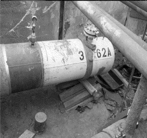
Test Headers and Exposed Pipe
