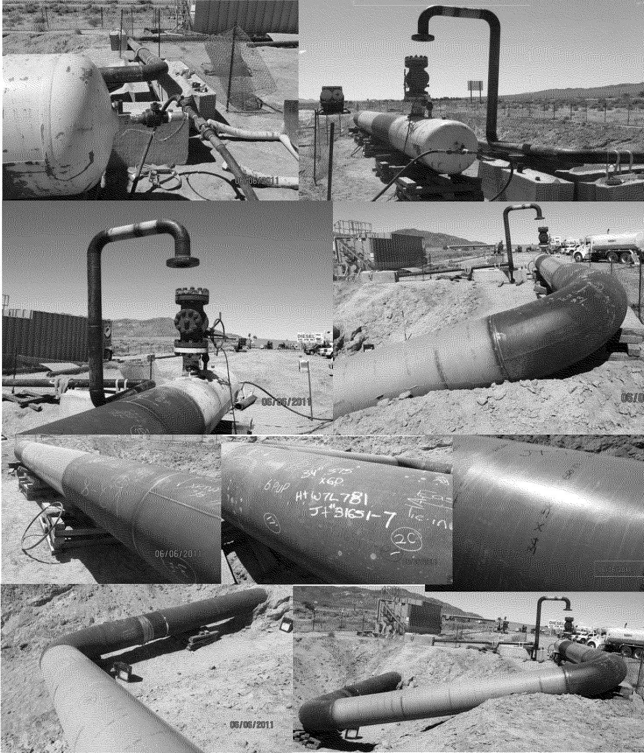
Test Header and Exposed Pipe Segments
