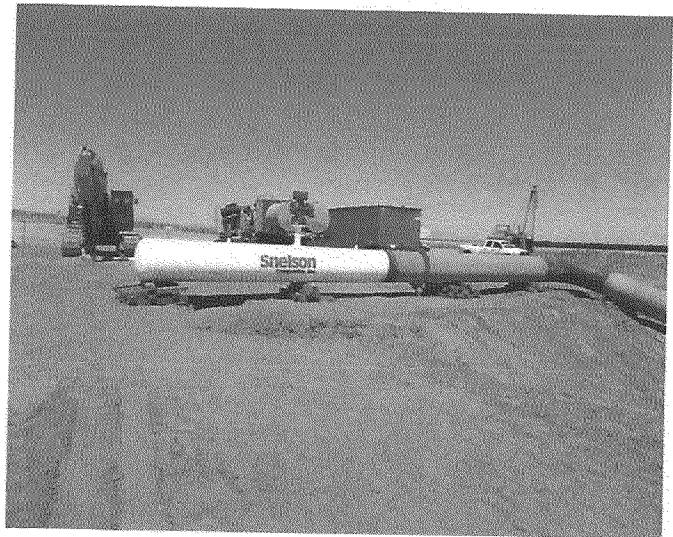
End of test segment header
