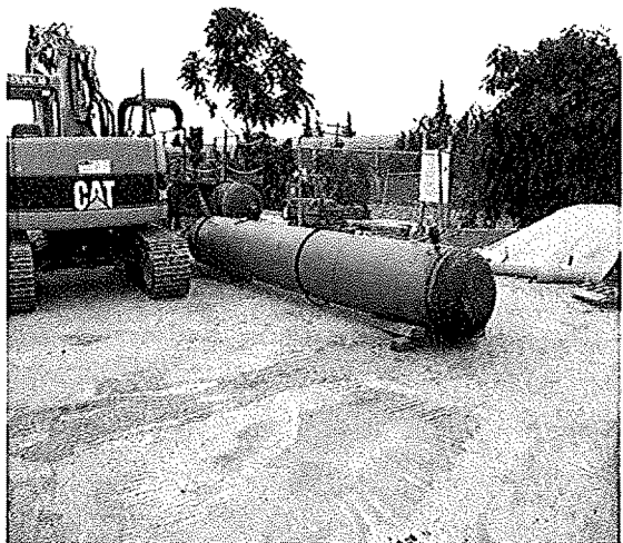
30" Tie-in pipe in test
