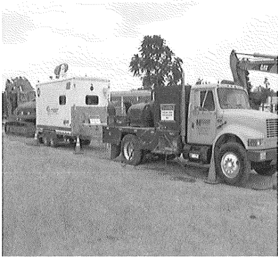
Test Pump and Trailer
