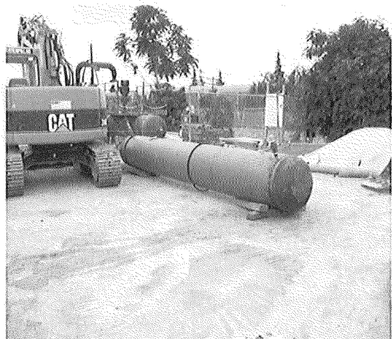
30" Tie-in pipe in test
