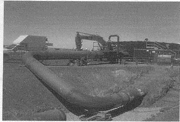
Test Header to Existing Pipe
