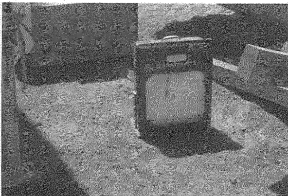
Restrained Temperature Chart Recorder in Ditch
