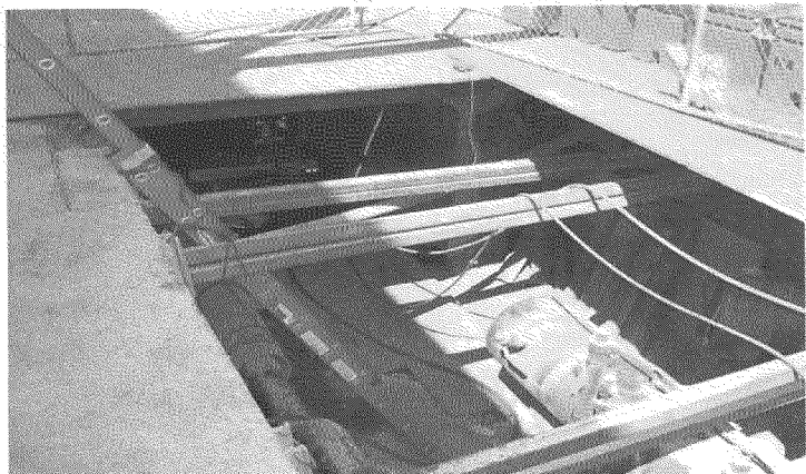
Trench to gain access to test header
