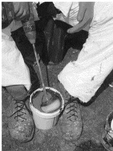
CAUTION: DO NOT use high speed mixing. DO NOT use solid multi bladed mixing paddles. High speed mixing will cause air bubbles to be trapped in the epoxy coating. This causes voids and pits in the pipe coating. Often the air pockets remain below the surface of the Protal.
