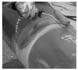
very difficult to maintain. A more reasonable range that you should be able to obtain is 20 – 60 mils. You should attempt to apply a single coat that is between 35-40 mil thick. If done carefully this will result in a coating between 20 and 60 mils.
