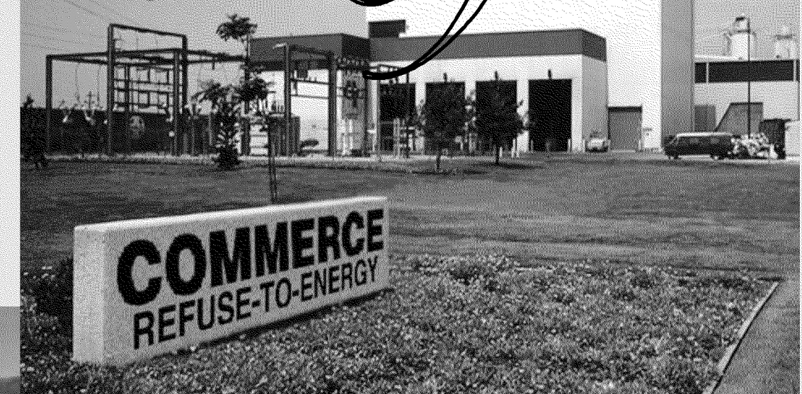
Commerce Refuse-to-Energy Facility, above, produces 10 MW of electricity from the burning of solid waste.
