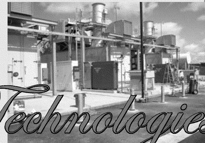
The Calabasas Landfill uses methane gas in combustion turbines. This plant is establishing new, lower air-emission standards.
