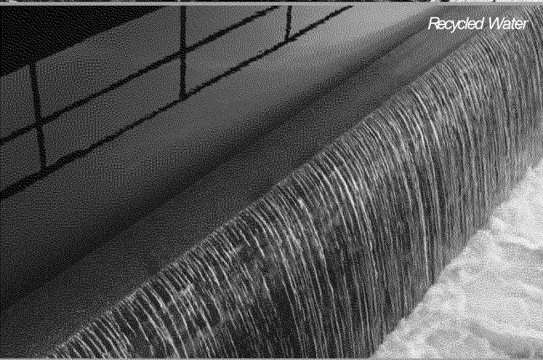
San Jose Creek Water Reclamation Plant
