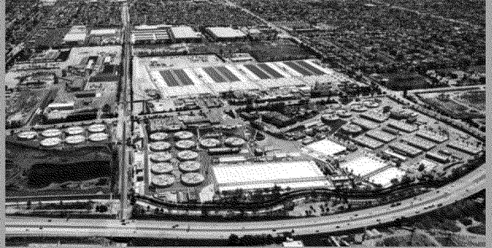
Joint Water Pollution Control Plant, Carson
