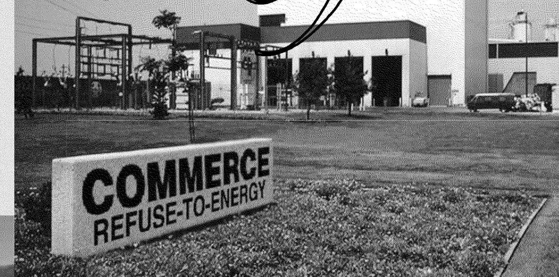
Commerce Refuse-to-Energy Facility, above, produces 10 MW of electricity from the burning of solid waste.
