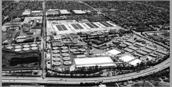
Joint Water Pollution Control Plant, Carson
