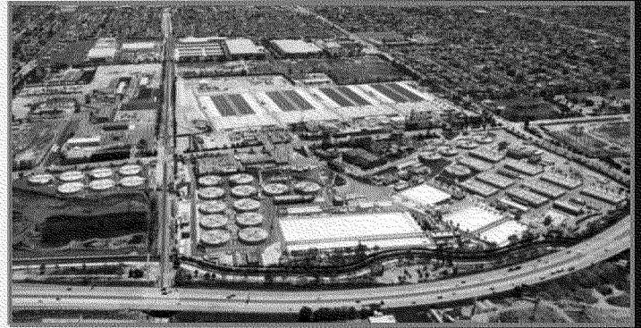
Joint Water Pollution Control Plant, Carson
