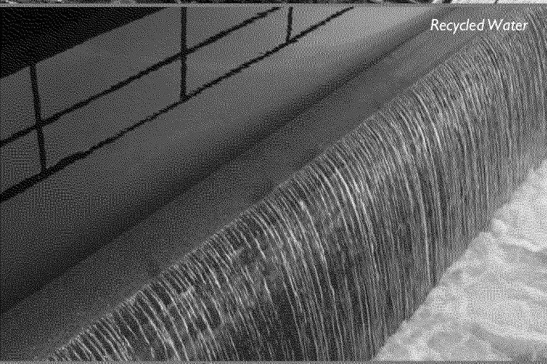
San Jose Creek Water Reclamation Plant
