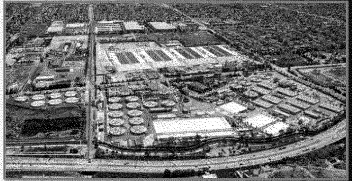
Joint Water Pollution Control Plant, Carson
