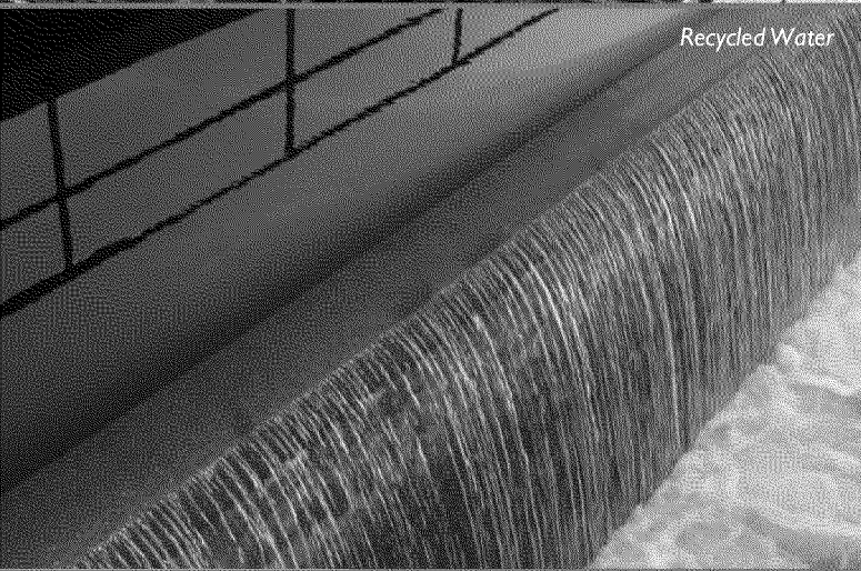
San Jose Creek Water Reclamation Plant
