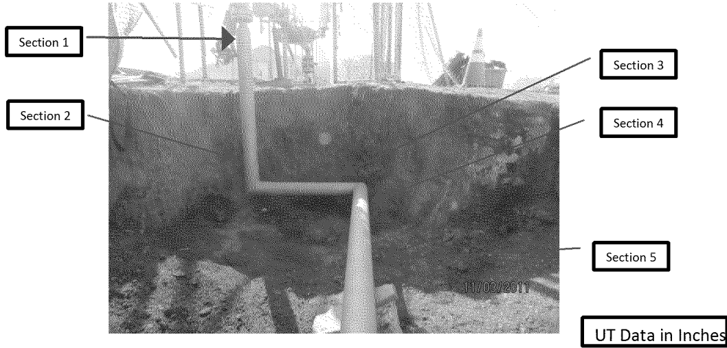
Clock position UT Data near welds
