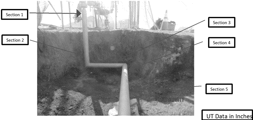
Clock position UT Data near welds
