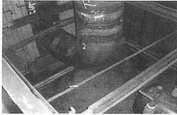
Test T-26 Test Head Tie In
