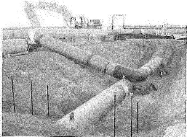
test head piping at location A, test 85
