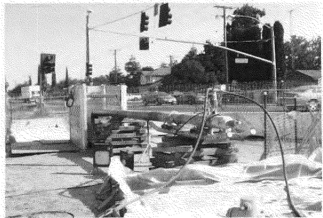
Tie In Pipe Test Head
