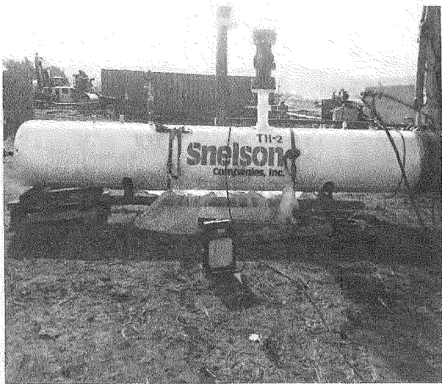
Test Headers & Pressure Recorder
