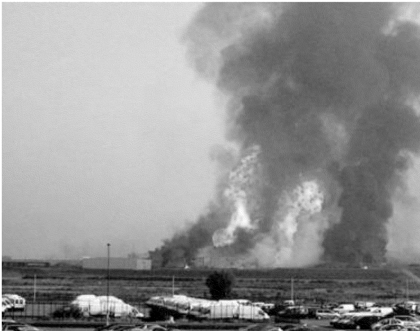
Photo 1 – Large diameter gas pipeline rupture
