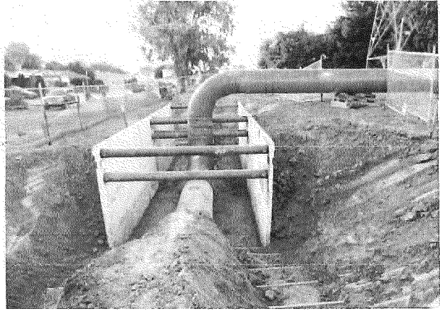
test 90C - excavation and risers at loc. B
