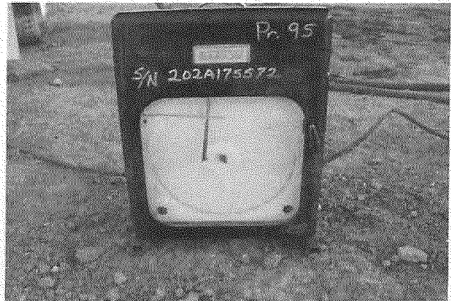
Test T-65A Pressure Gauge
