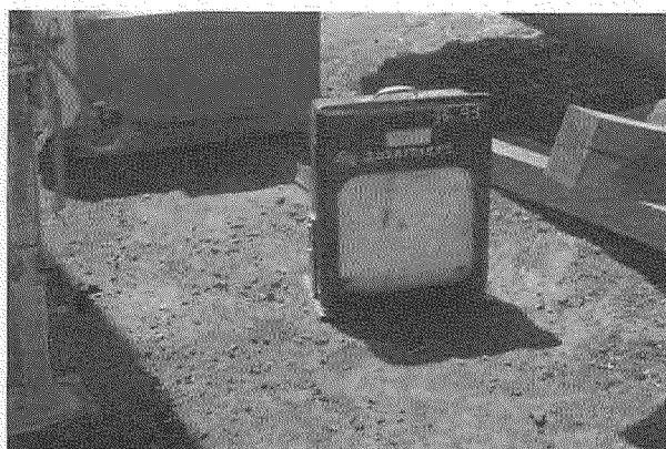
Restrained Temperature Chart Recorder in Ditch
