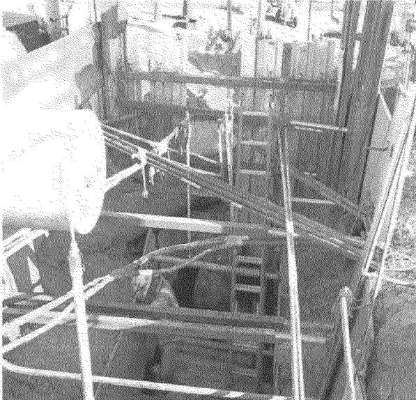
24" Transmission Line Tie-in
