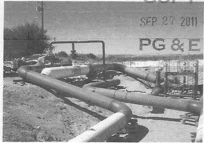
test 56 Loc.B testhead on 34" mainline
