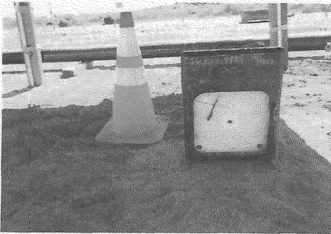
Test 56 loc.A remote pipe temp. recorder
