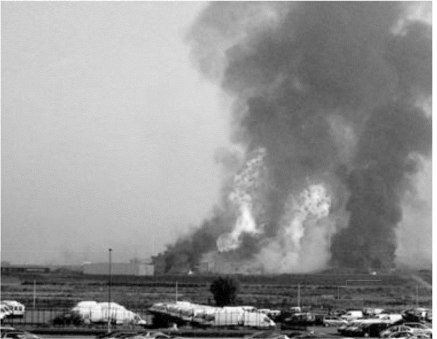
Photo 1 – Large diameter gas pipeline rupture
