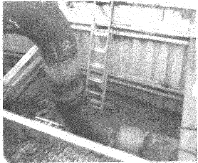
Test Head Tie-In to Mainline.
