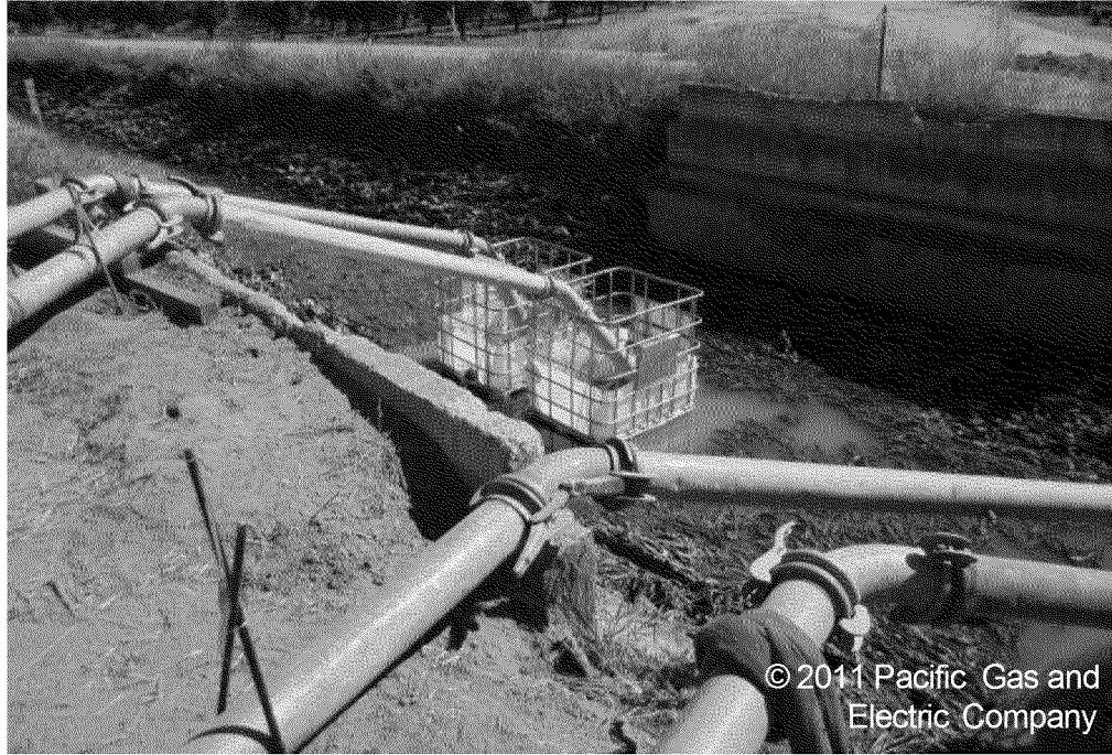
Water disposal in a drainage/irrigation canal
