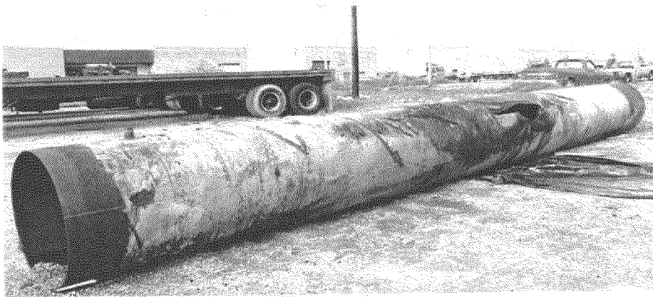
Overall View of the Piece Removed
