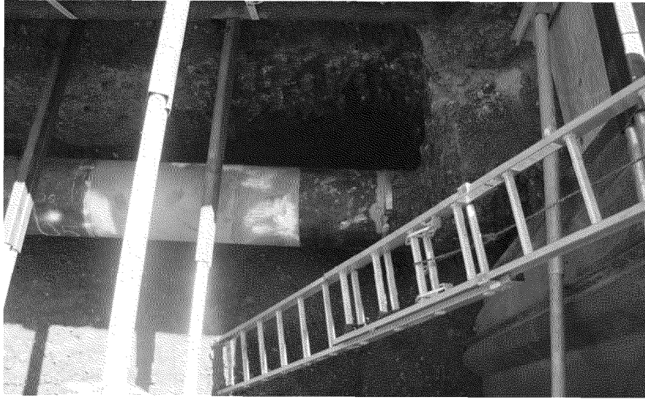
Overview of Dig Site DS after Additional coating removed
