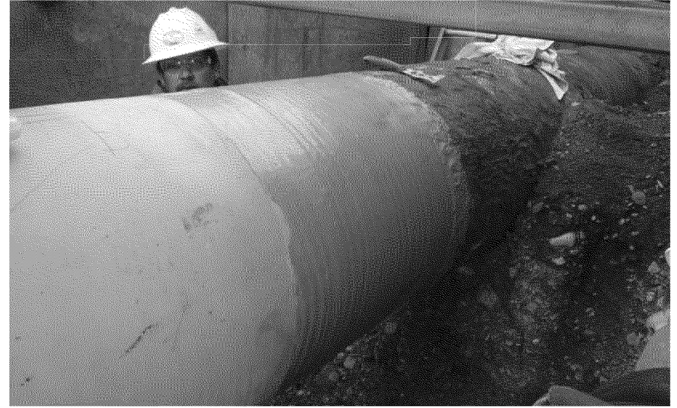
Overview of final coating condition US 9:00
