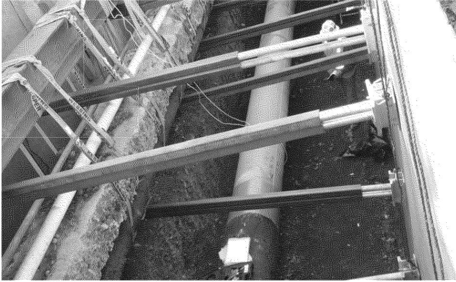
Overview of final coating condition
