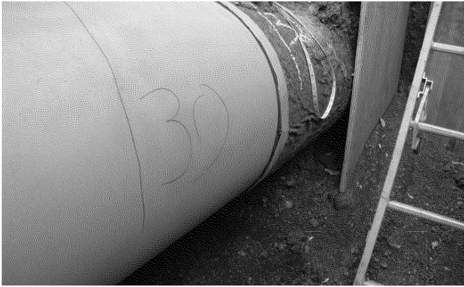
Overview of coating condition 30 ft to 33 ft, 3:00 position
