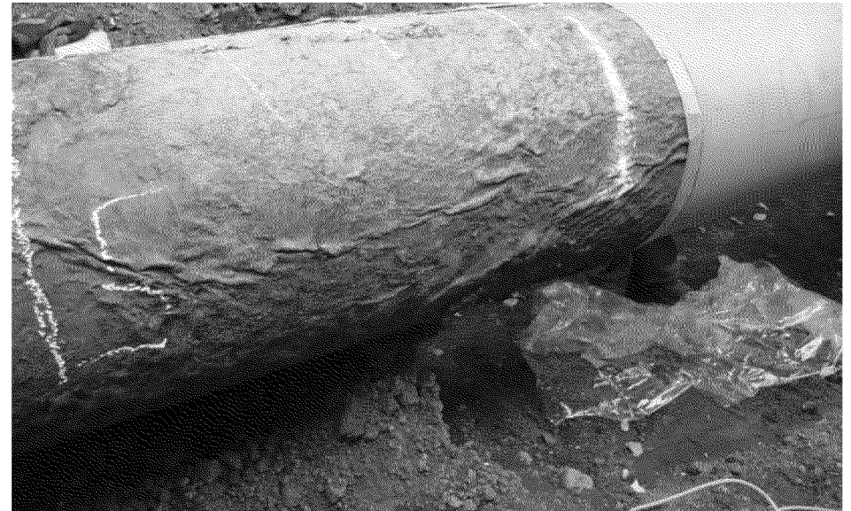
Overview of coating condition 5 ft to 10 ft, 3:00 position
