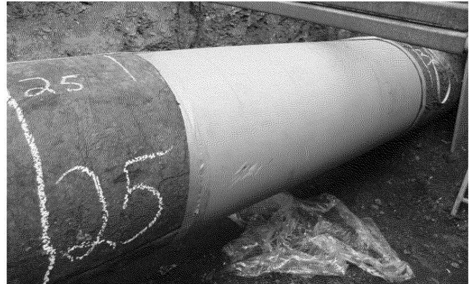
Overview of coating condition 25 ft to 30 ft, 3:00 position
