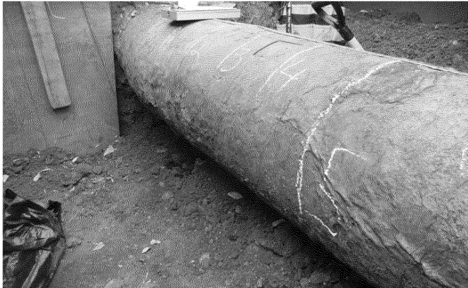
Overview of coating condition 0 ft to 5 ft, 3:00 position
