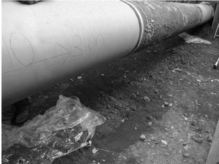
Overview of coating condition 10 ft to 15 ft, 3:00 position
