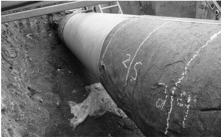
Overview of coating condition 20 ft to 25 ft, 9:00 position
