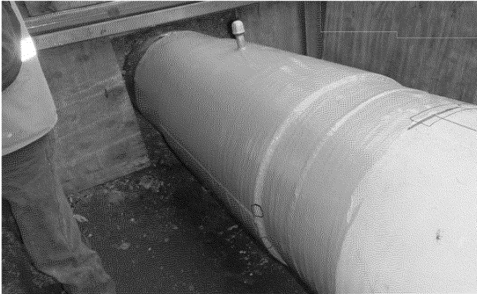
Overview of final coating condition DS 9:00
