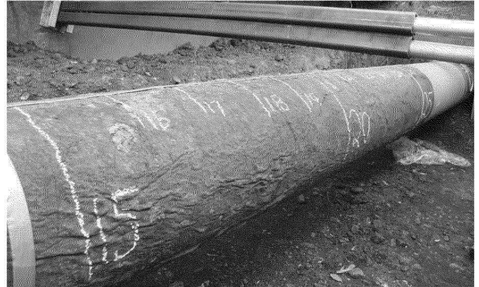
Overview of coating condition 15 ft to 20 ft, 3:00 position
