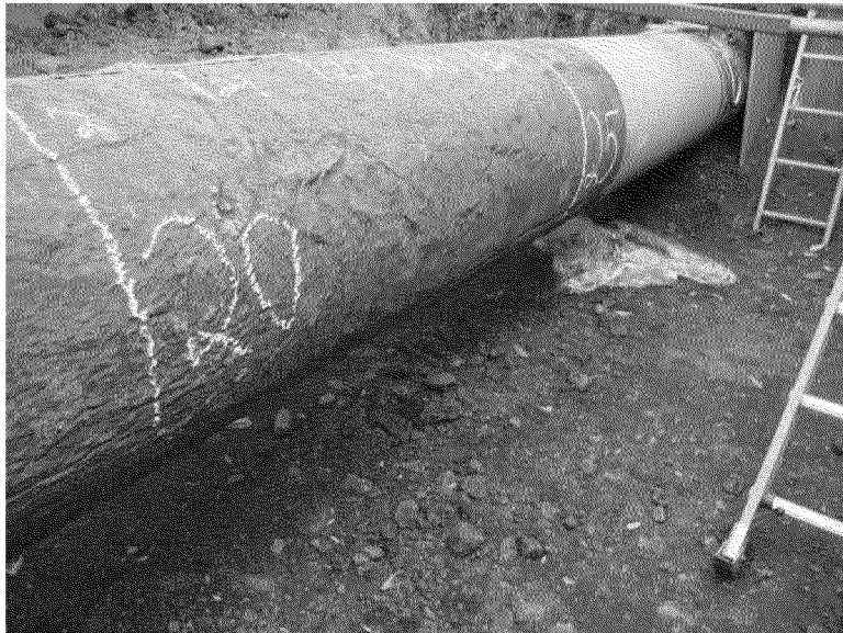
Overview of coating condition 20 ft to 25 ft, 3:00 position
