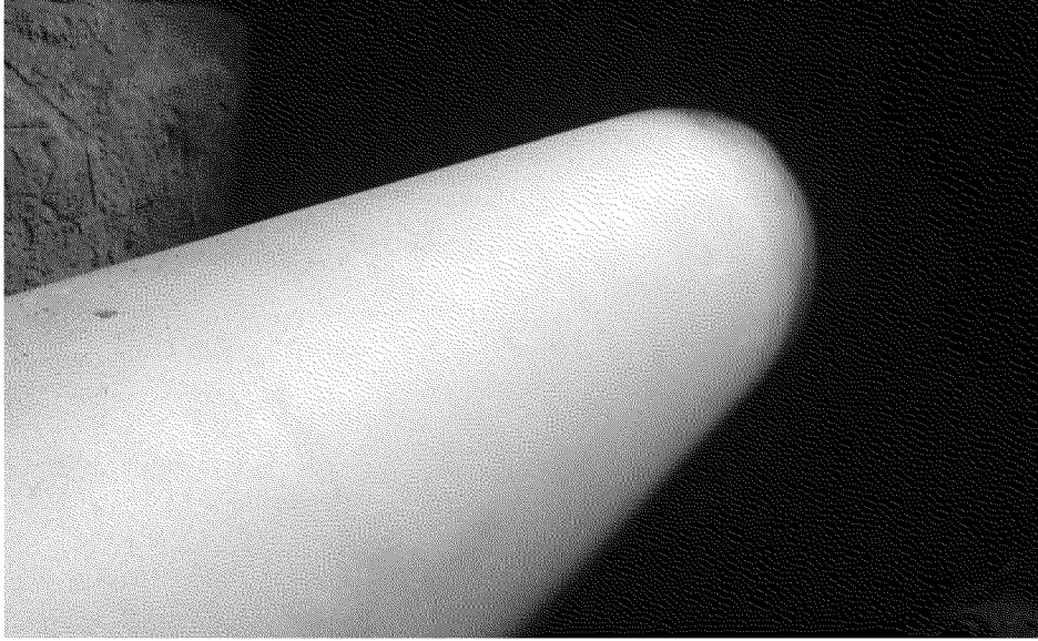
Overview of clean blasted inspection area prior to repair activities
