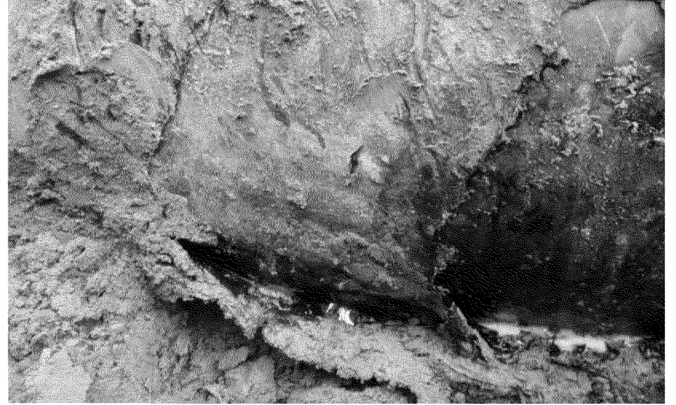
Close up of removed coating to find leak
