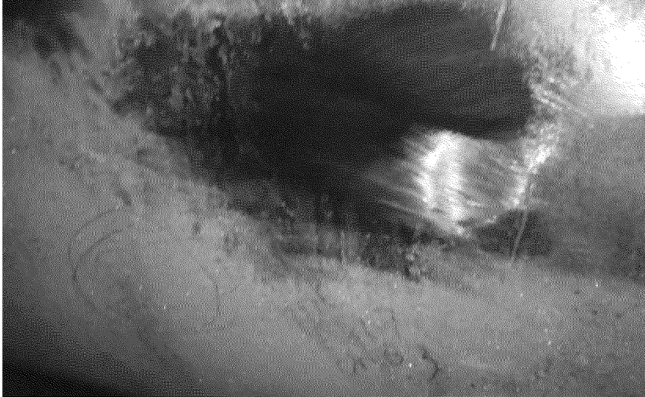
Overview post grind (MPIOK) of LIN-04
