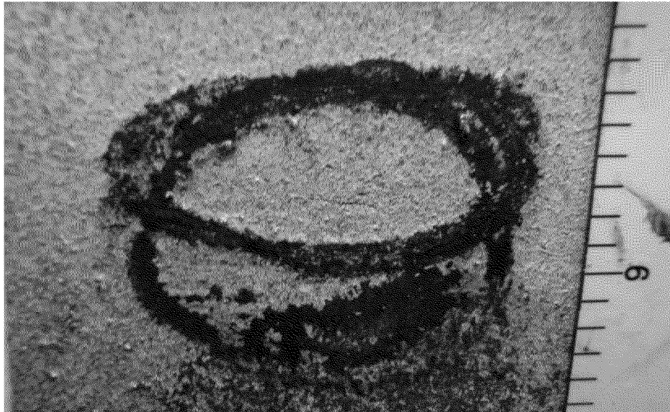
Close up of second inspection MT Indications of LIN-06
