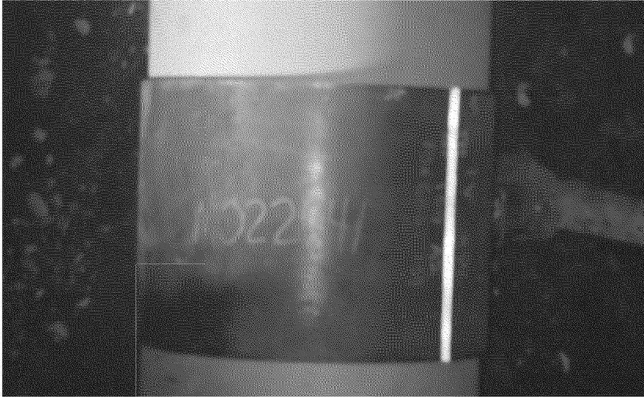
Overview of full encirclement sleeve "B" placement
