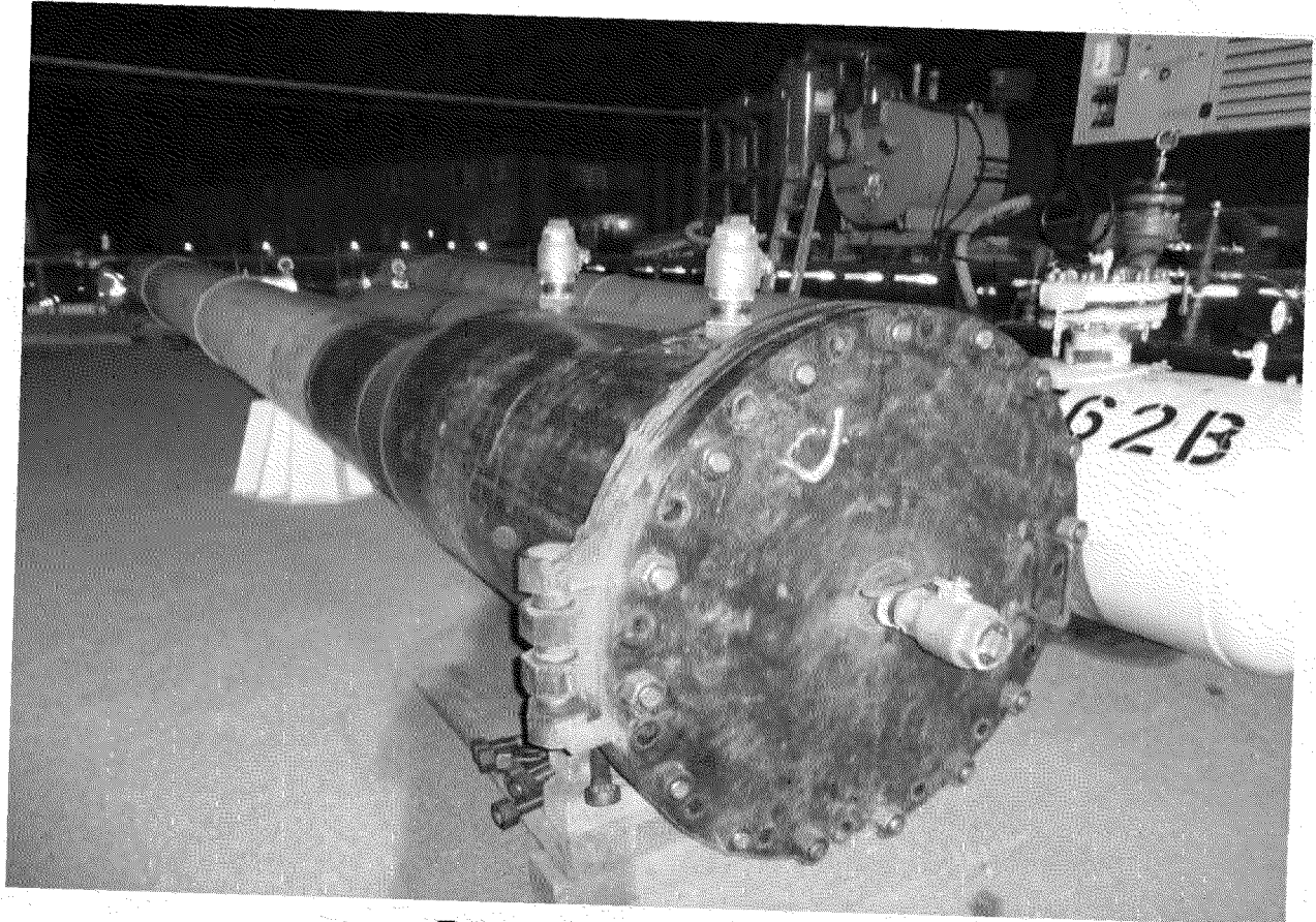
Exposed Pipe and Test Header
