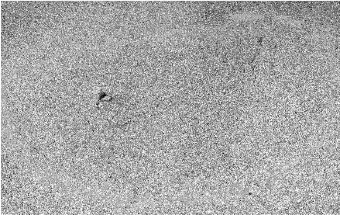
Figure 37. Surface Imperfection, T117-CE-LS-W
