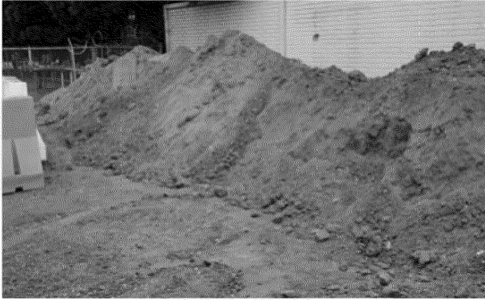
Overview of spoil pile
