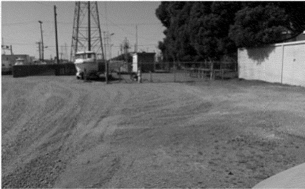
Overview of completed cover looking downstream
