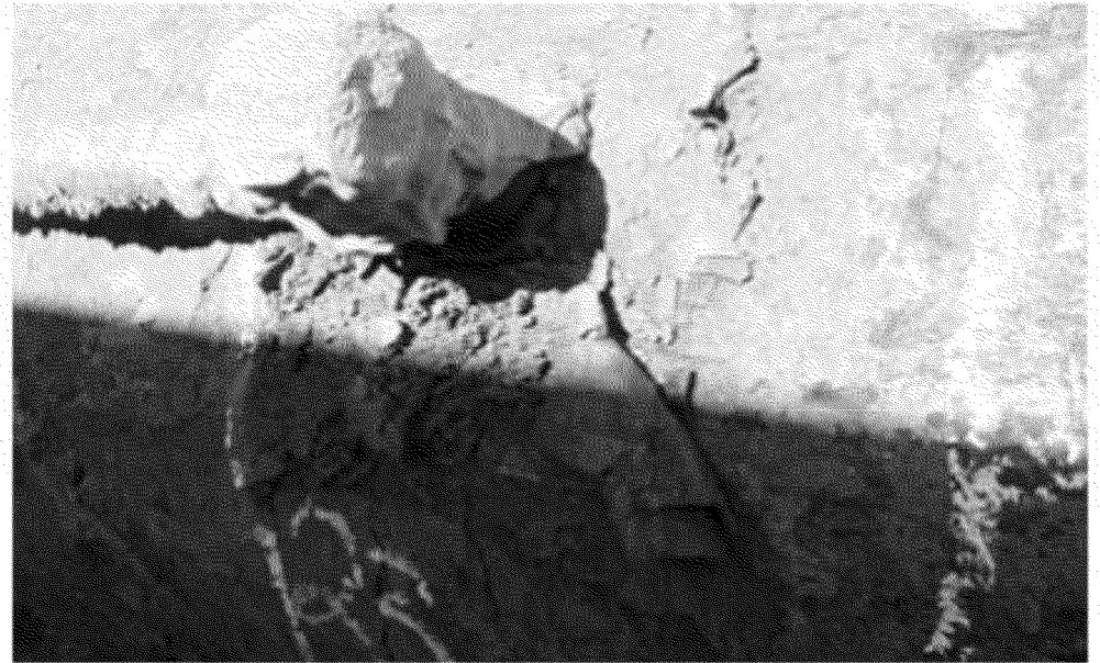
Overview of coating condition @ 12:00 position
