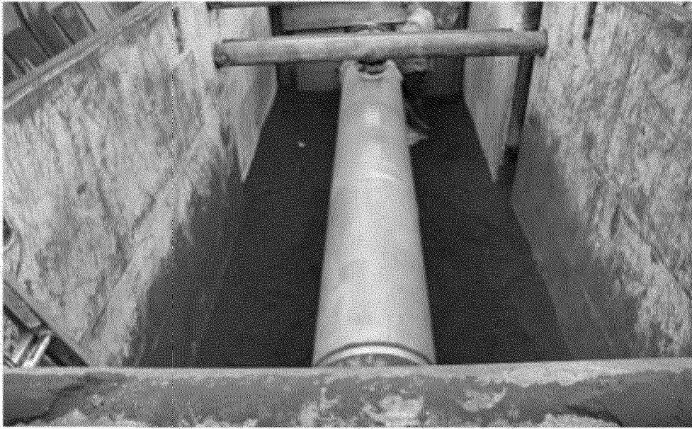
Overview of Dig Site T47-L153-C
