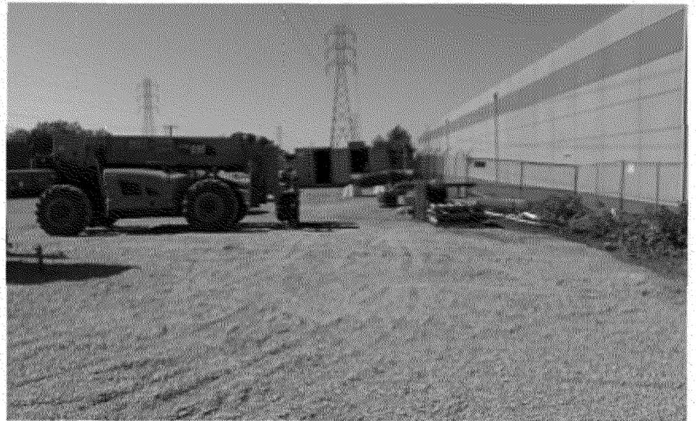
Overview of completed cover looking downstream
