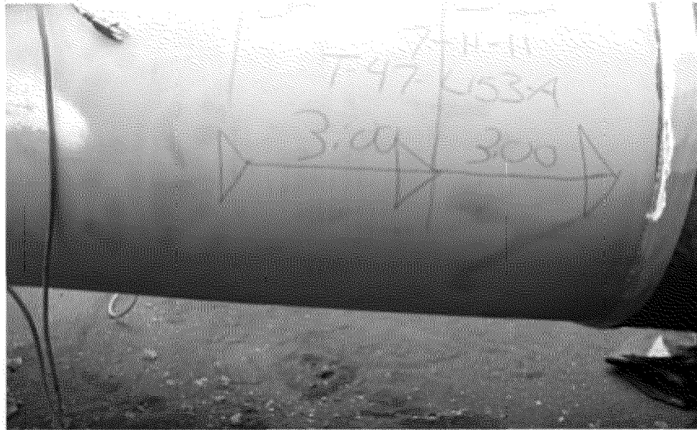
MPI area extended to 34ft due to lamination in cut line area
