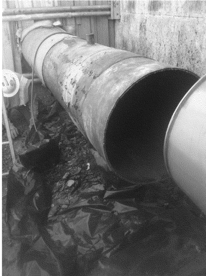
5 6 7 8 9 10 11 12 13 14 15 16 17 18 19 20 21 Illustration C: Coating Deficiencies
