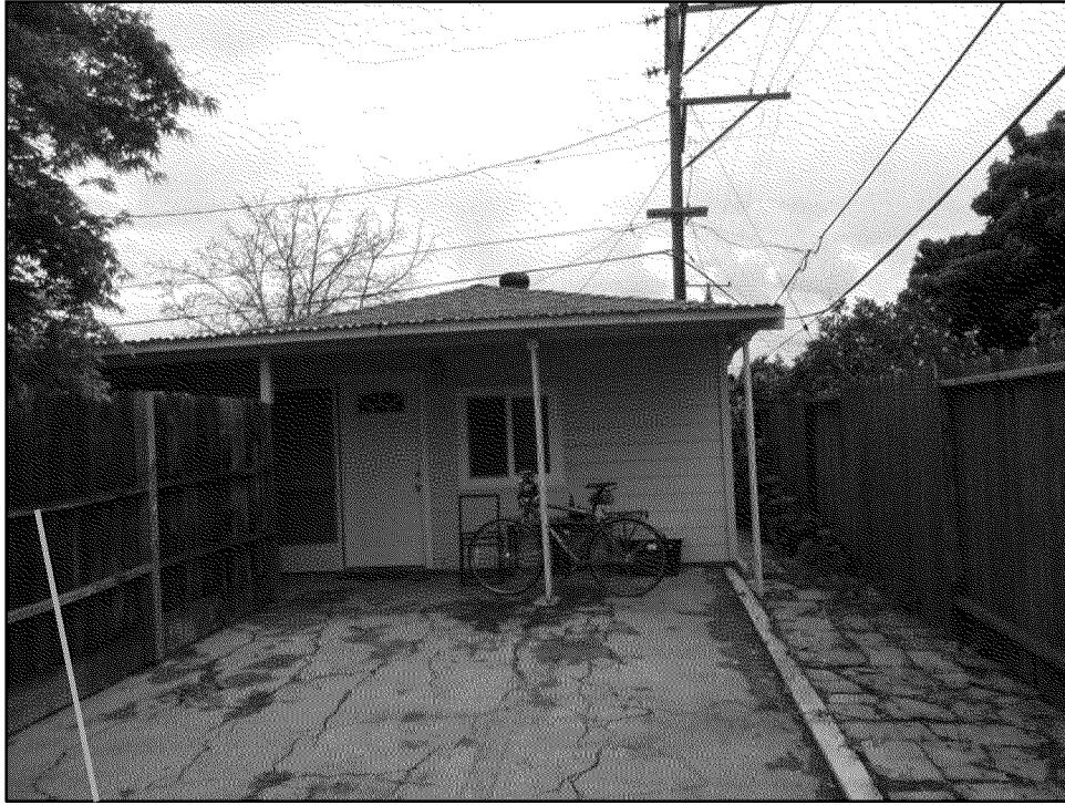
Second House (expanded garage) Overhang within the easement and over the pipe.
