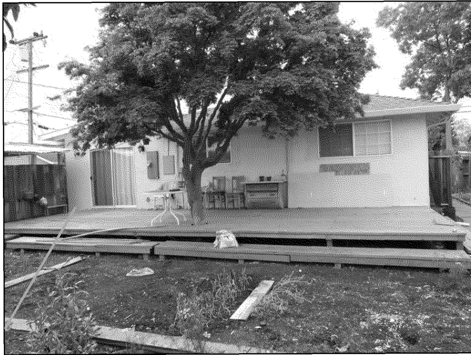
Main House is over the line.
