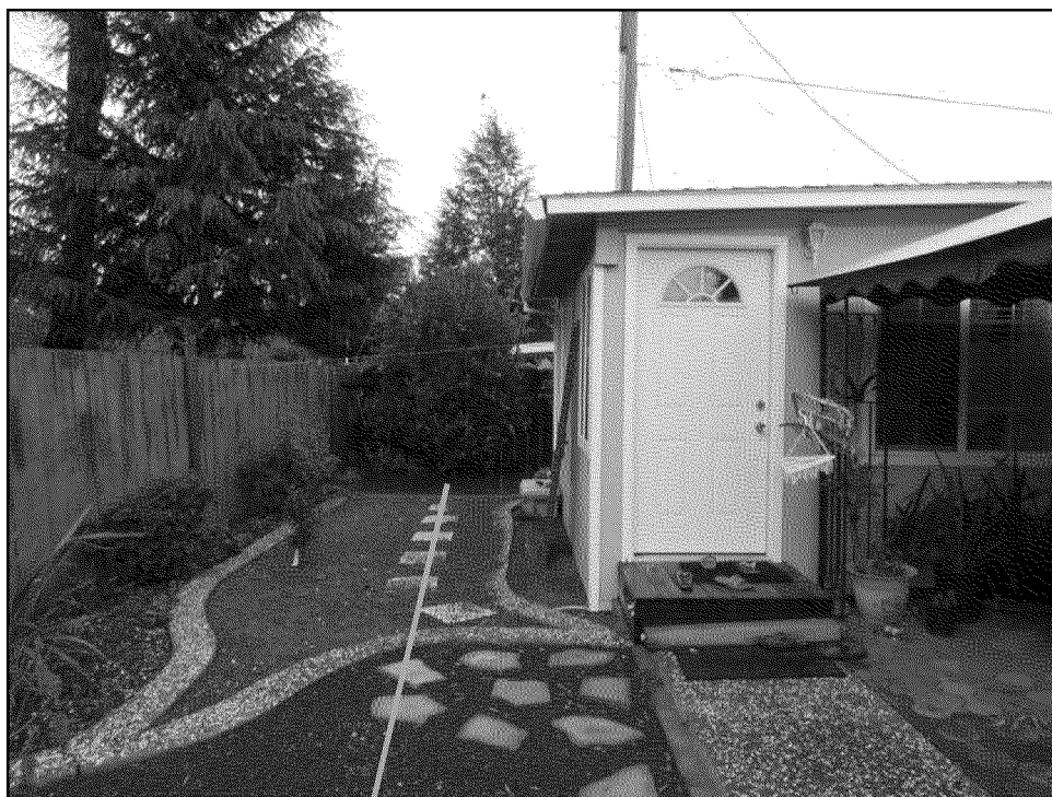
House, is within the easement area by 1.4'.
