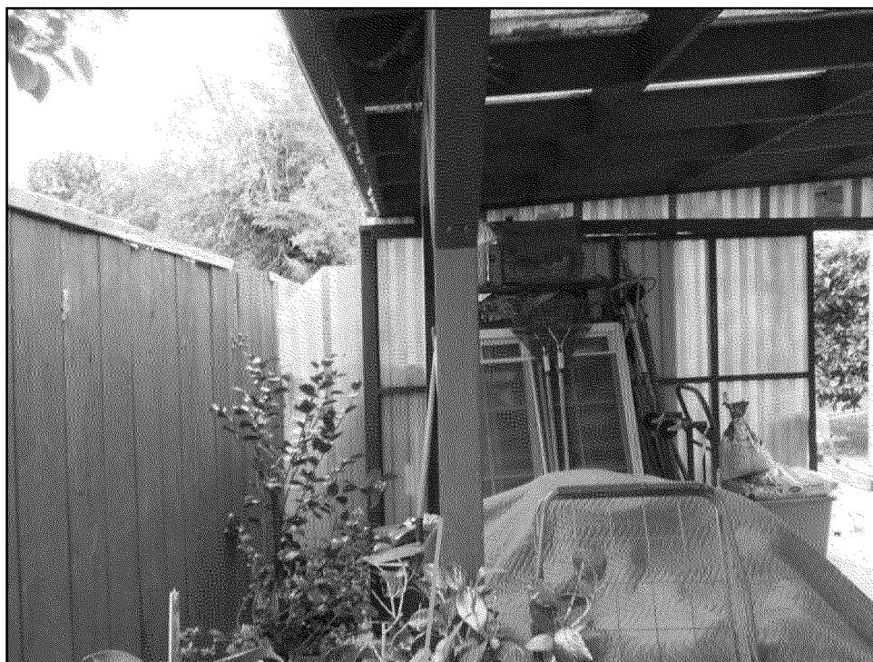
Standing on the line looking west from the covered patio
