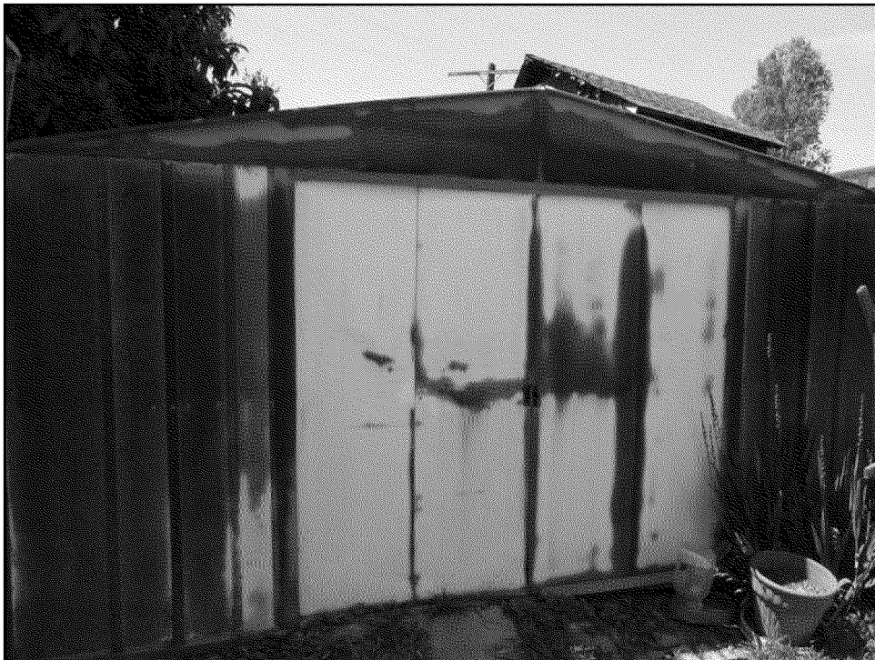
Shed within the easement area.
