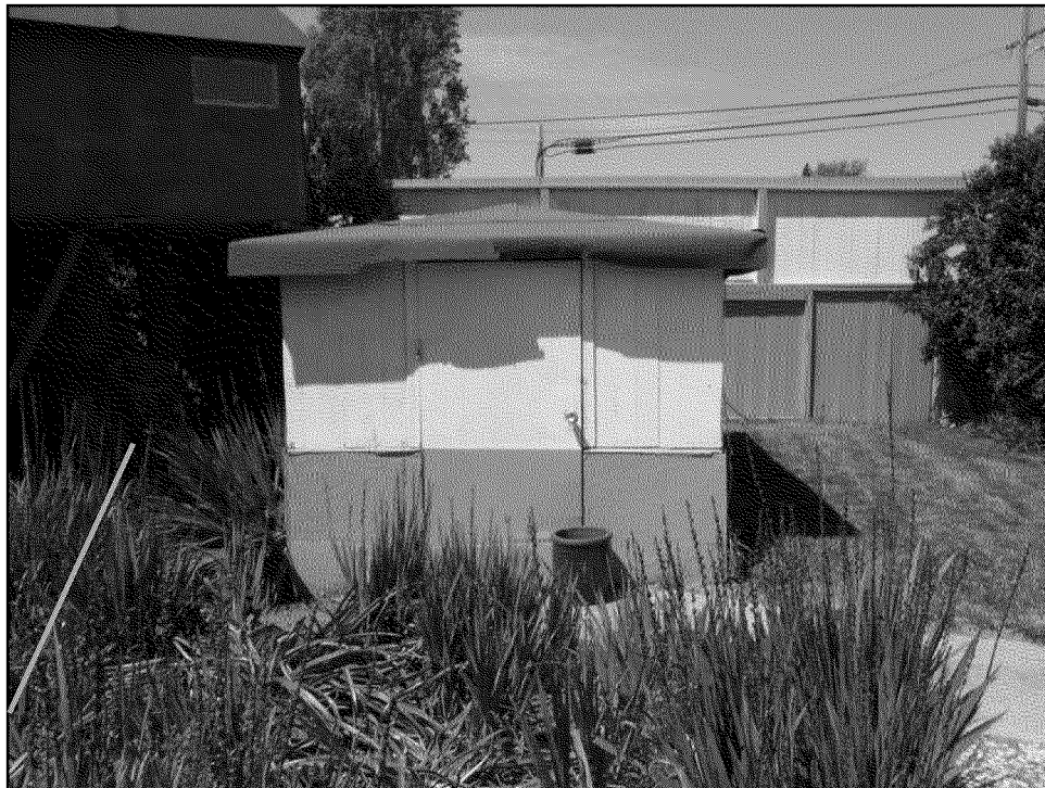
Shed within the easement area.
