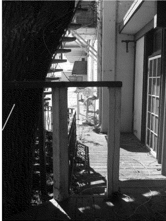
Standing to the right of the line looking southwest through the office building
