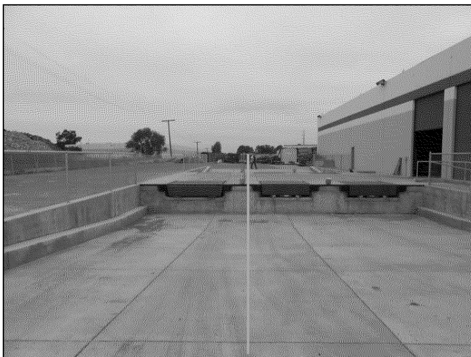
Standing on the line looking to the south.
