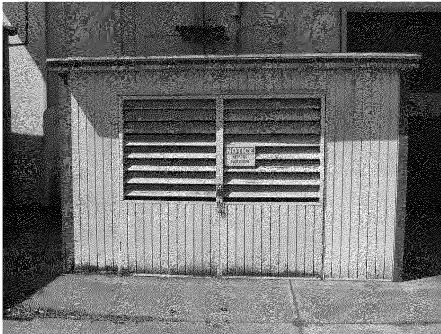
Standing on the line looking at the first shed
