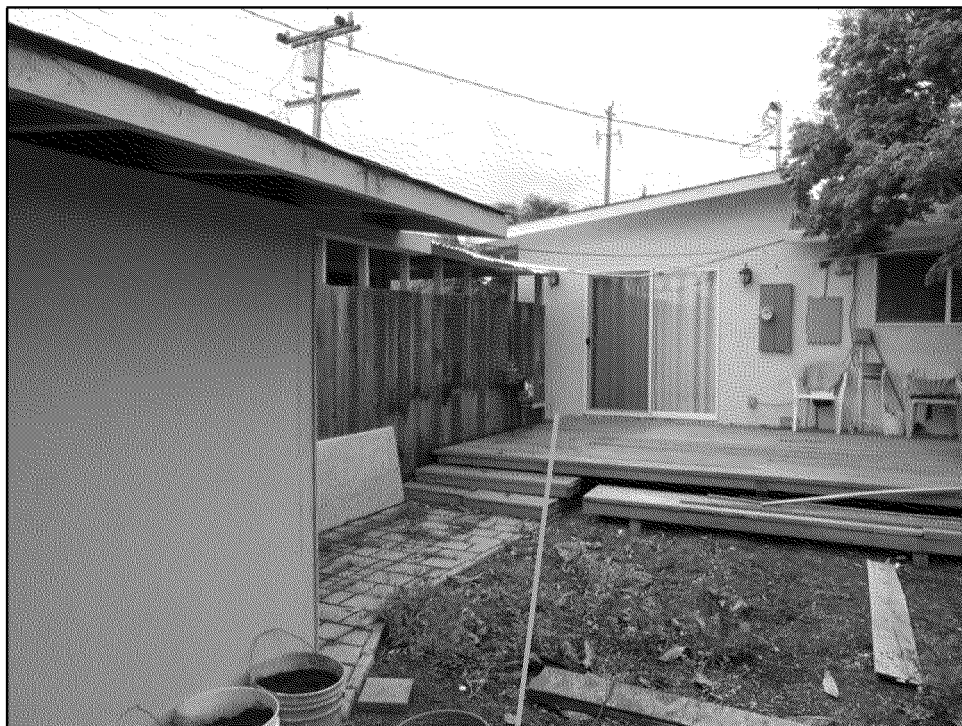
Standing on the line looking west.
