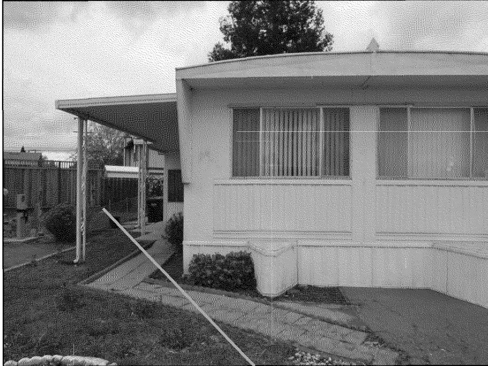
Standing on the line looking west.
