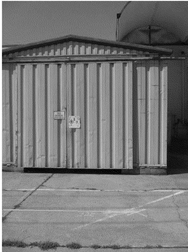
Standing behind the line looking at the shed
