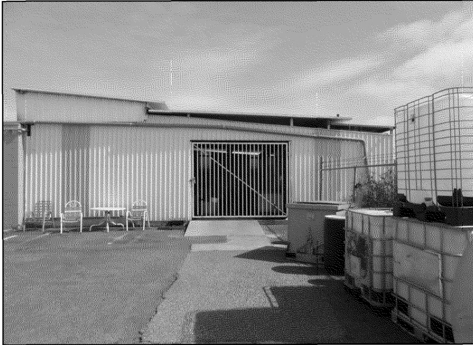
Building is over the line.
