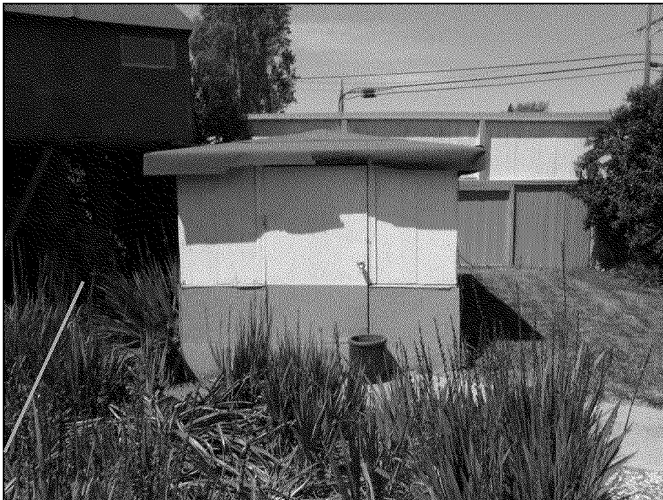
Shed within the easement area.
