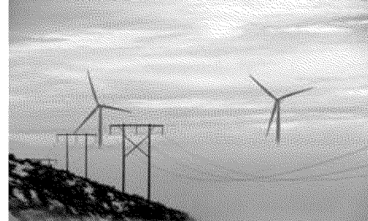
BPA's transmission lines continue to play vital role in developing wind power.
