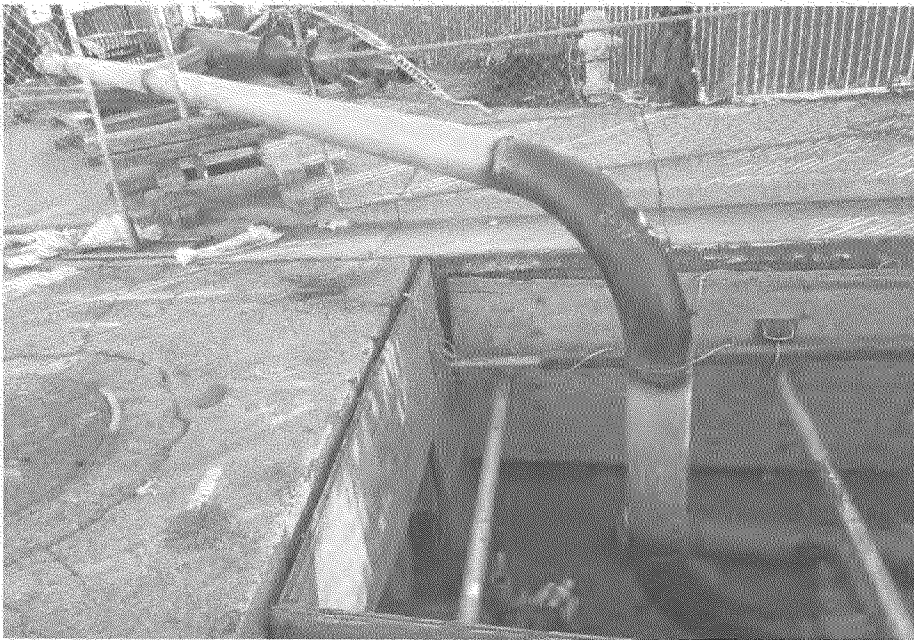
Test 102F-12 Loc. B riser and test head
