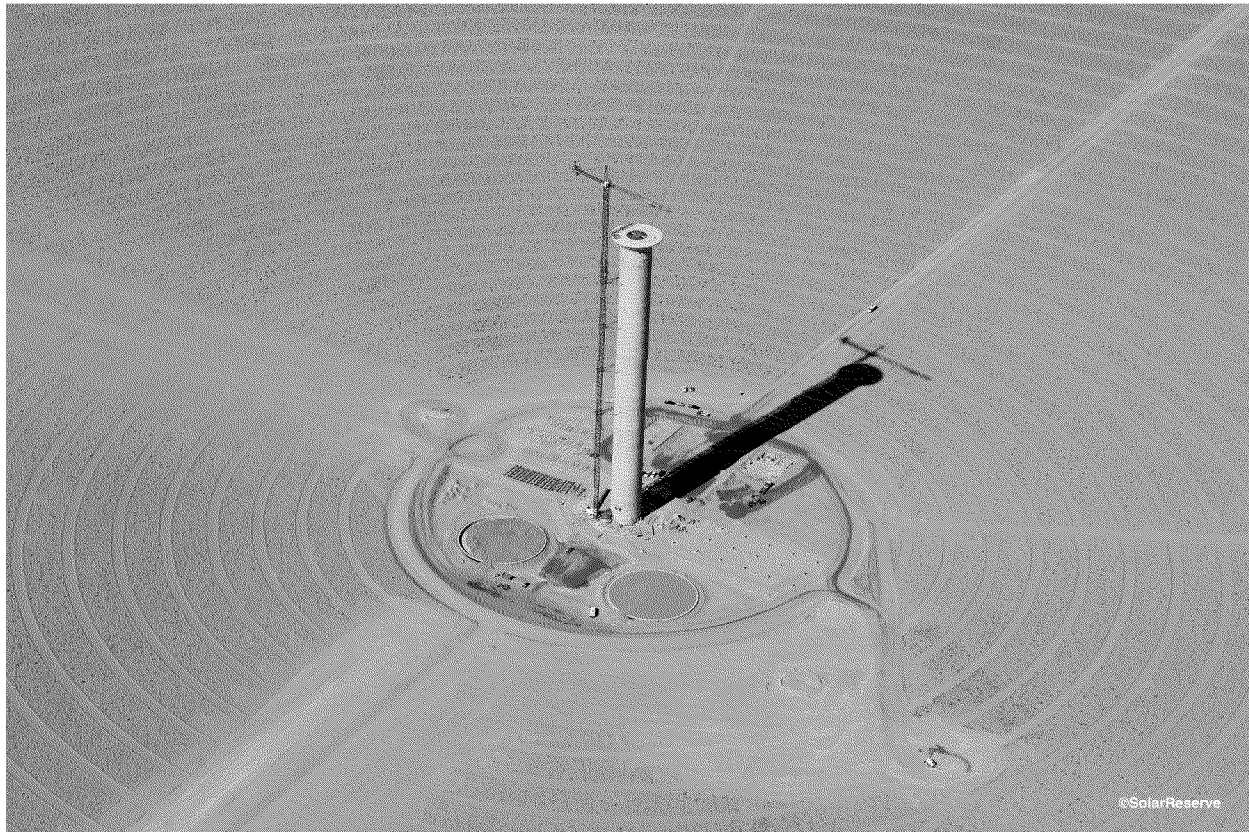
Figure 2 - Crescent Dunes project under construction near Tonopah, NV
