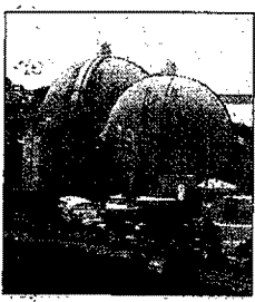
THE REGISTER San Onofre nuclear power plant.
