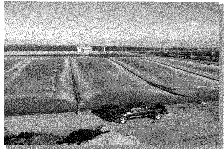
Operating Digester, Generation Facility and Background
